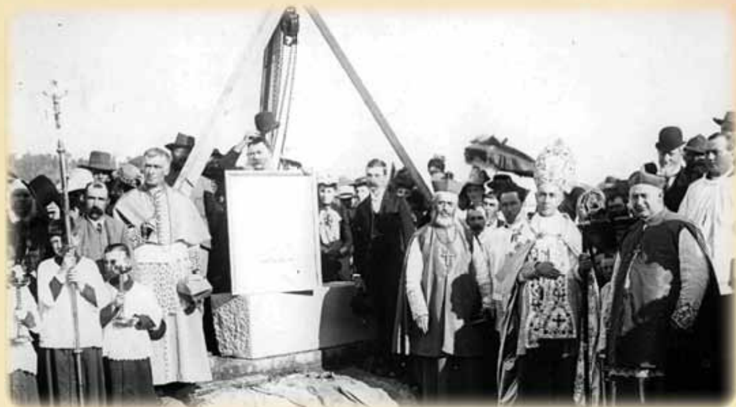
Laying of the Foundation Stone of St Carthage's Cathedral, 4th October, 1892. Bishop Jeremiah Doyle stands to the left. On the right the three prelates are Bishop James Corbett of Sale, Cardinal Patrick Moran, Sydney and Archbishop Thomas Carr, Melbourne. Wardell's framed perspective view rests on the stone.
