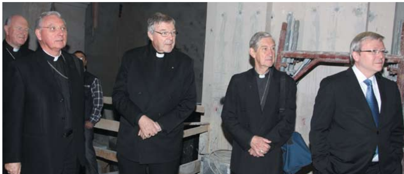
L-R: Archbishop Hart, Bishop Jarrett, Cardinal Pell, Archbishop Hickey and Mr Kevin Rudd inspect progress on the renovations (Image from Kerry Myers)
